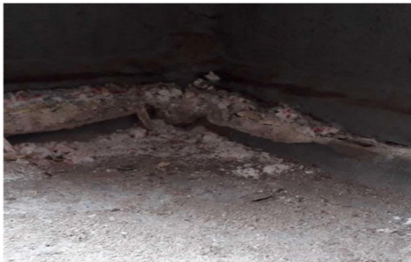
Figure 13. Crack in the port-side (Br) heat shield of the Meteoro
