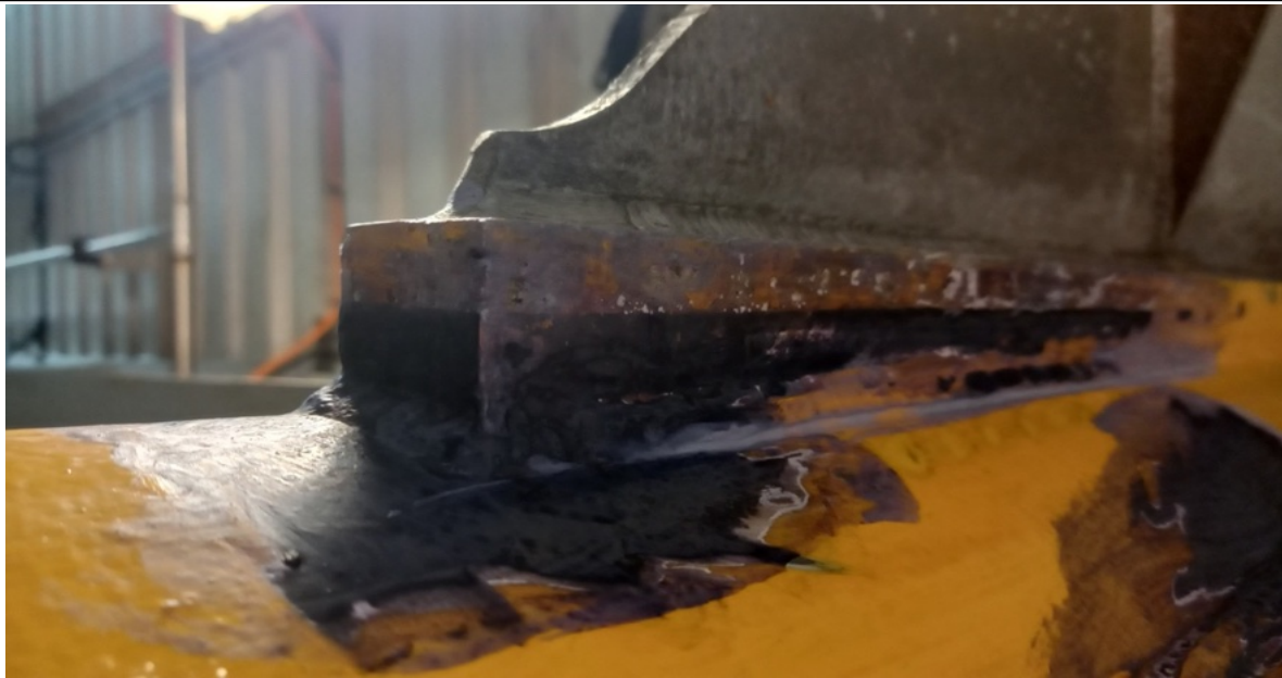
Figure 12. Unscheduled repainting job with Open-Air Transition-Joints (Condor)
