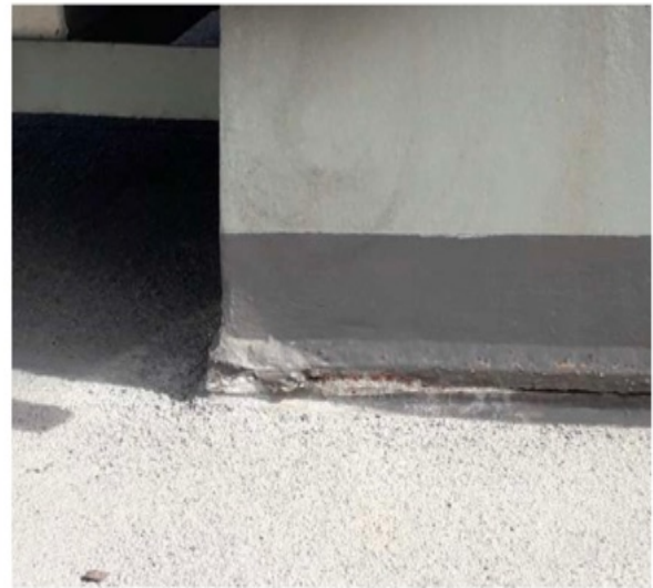
Figure 9. Crack in the startboard-side (Er) heat shield of the Rayo
