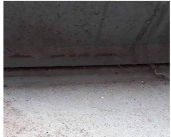
Figure 7. Crack in the port-side (Br) heat shield of the Meteoro
