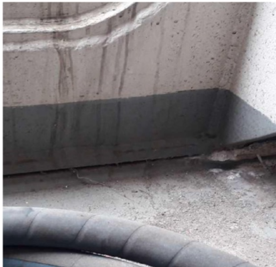
Figure 8. Crack in the port-side (Br) heat shield of the Meteoro
