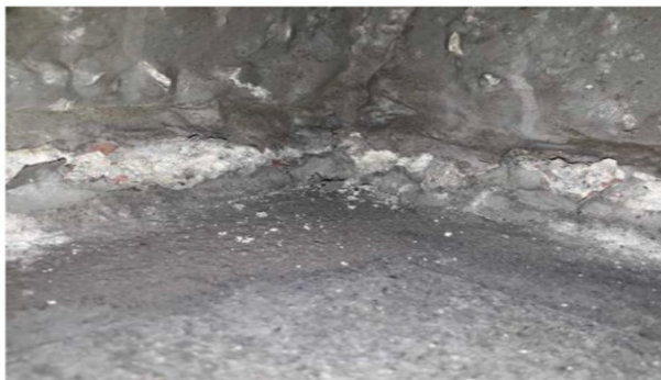
Figure 15. Corner of the port-side (Br) heat shield of the Relámpago
